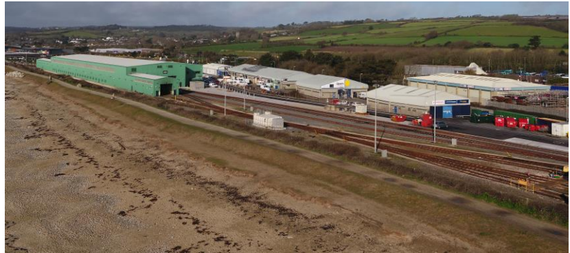
Photo Prior To Construction Works, March 2019 (Kemp Engineering)
