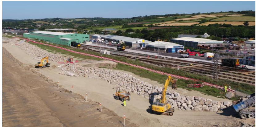
Photo During Construction Works, July 2019 (Kemp Engineering)
