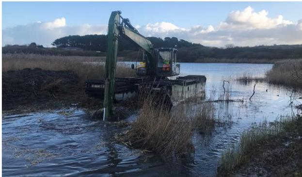
An amphibious excavator is being used for the reed clearance and construction of the deep-water channels. It can track on solid and semi solid ground as well as floating on water. It is operated with bio-oil and is adapted to work in environmentally sensitive areas such as Marazion Marsh.
