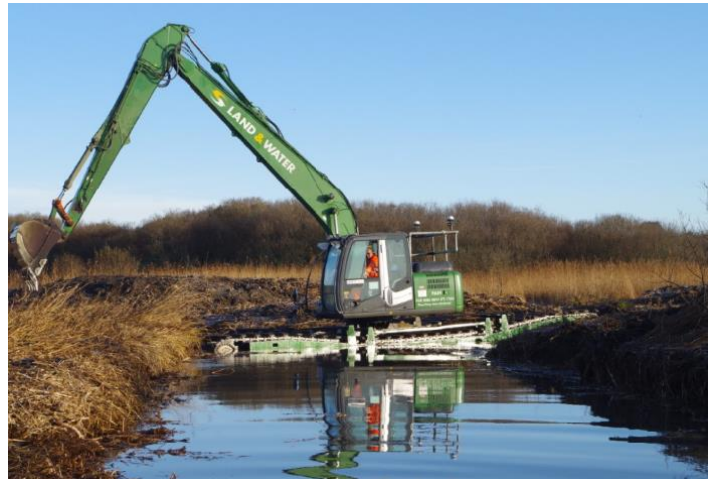
2 nd December 2019: Amphibious excavator creating open water channels
