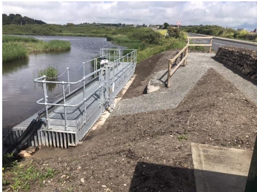
Photo Post Completion, June 2020
