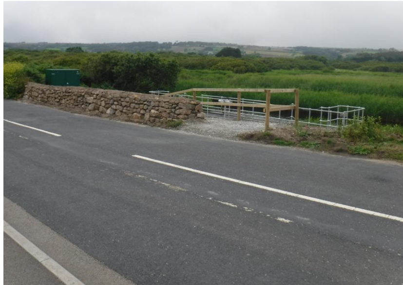
Photo Post Completion: View From The Road, June 2020
